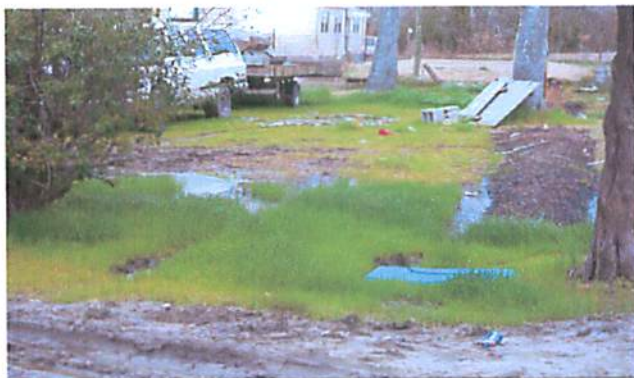
Signs of a failing septic system
